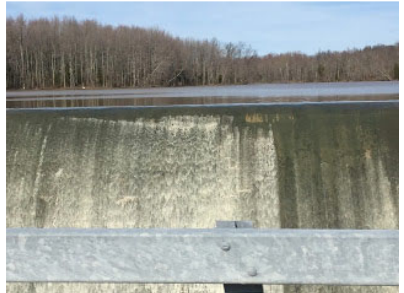
Stonelick Lake Dam
