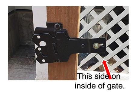
On the outside of the fence, the latch must be placed no less than 54" above grade.
